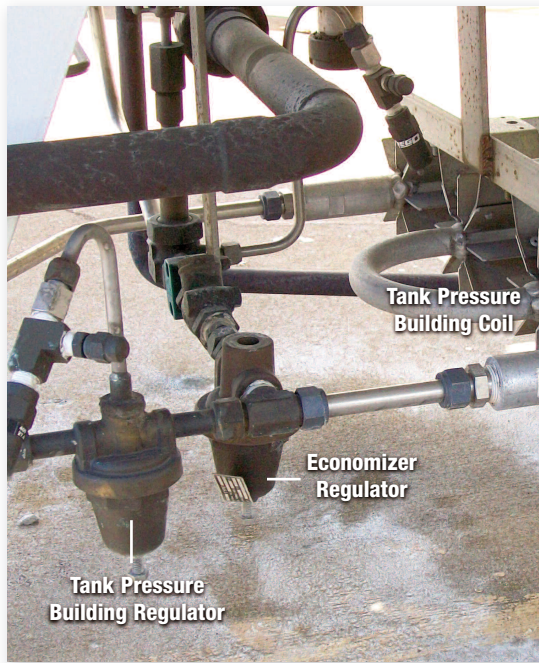
Figure 9: Tank Pressure Control System
